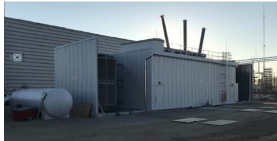
Transformer and shunt reactor hall
