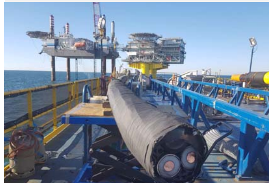
One of the two KF CGS AC sea cables (150kV) during installation campaign in front of KFB platform.
